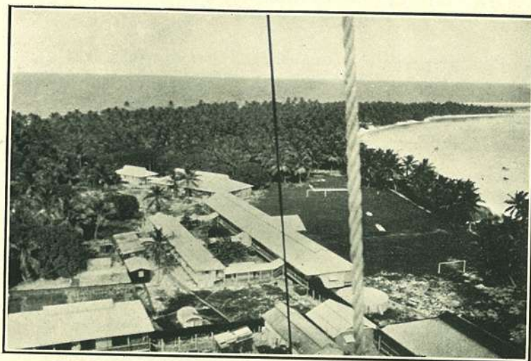
A VIEW OF THE CABLE STATION TAKEN FROM THE WIRELESS MAST.
