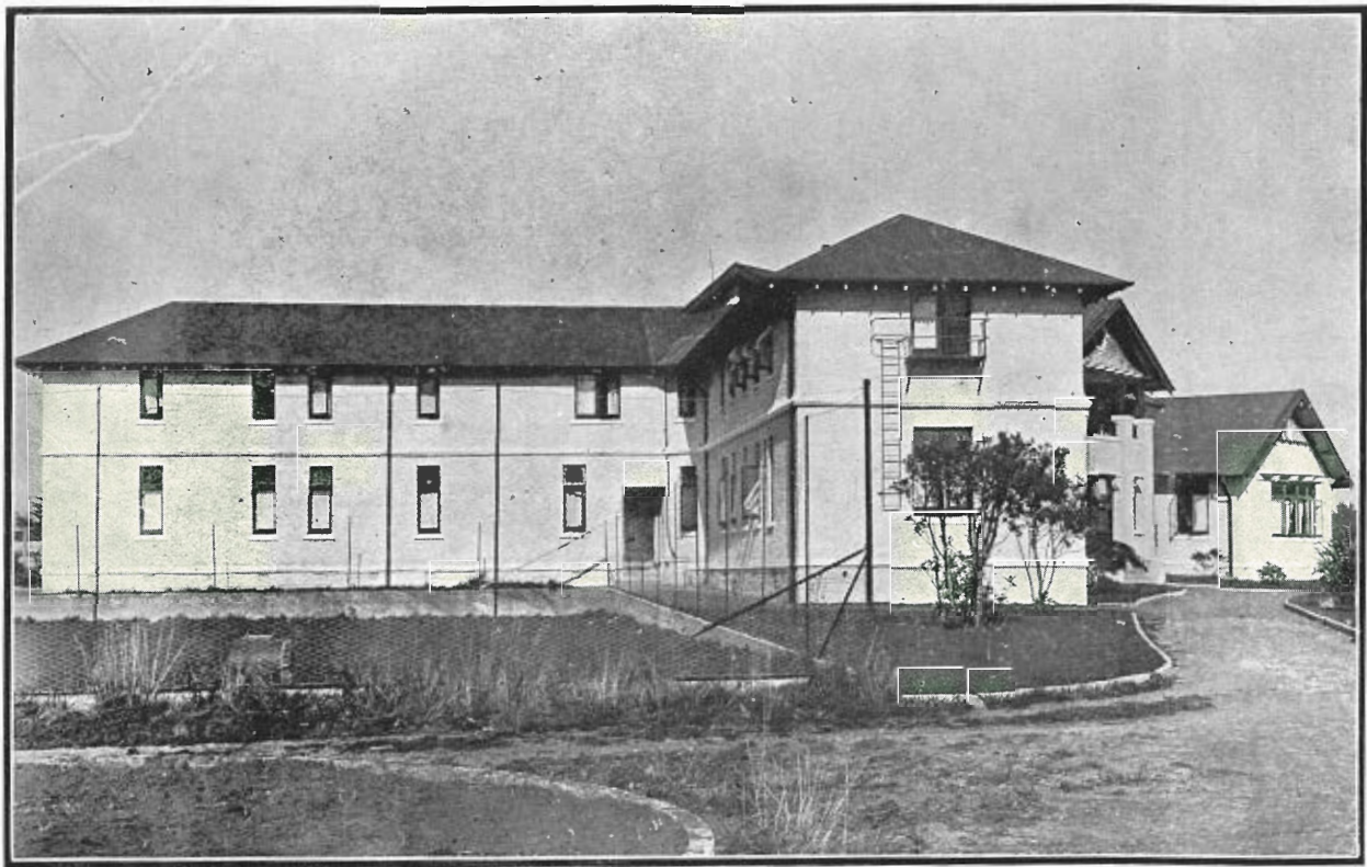
BOARDING BLOCK. (SHOWING NEW WING.)
