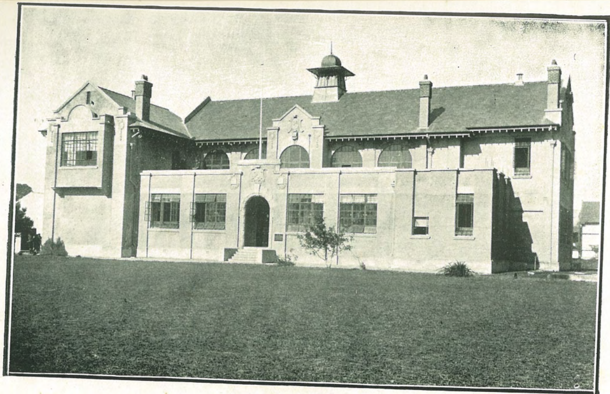
FRONT VIEW OF SCHOOL.
