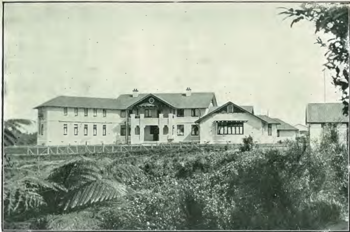
NEW HOUSE FROM ACROSS THE GULLY.
