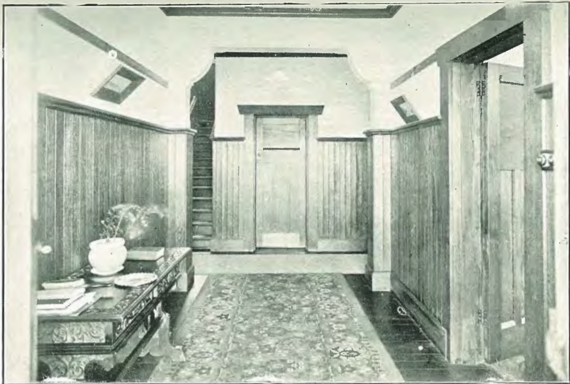
FRONT HALL : NEW BUILDING.
