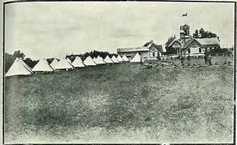
WORK IN CAMP.
