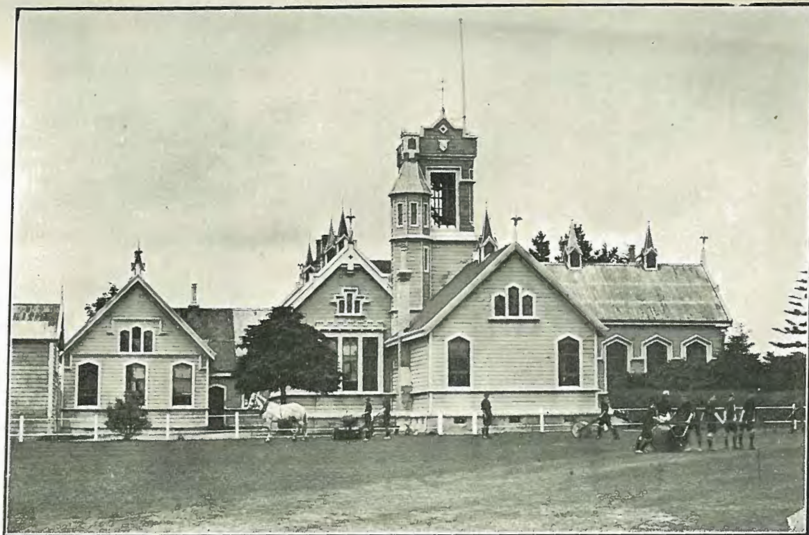
WORK ON THE CRICKET GROUND.
