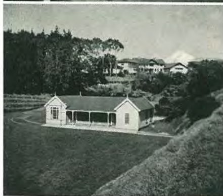
PRIDHAM HOUSE. VIEW FROM TERRACES.
