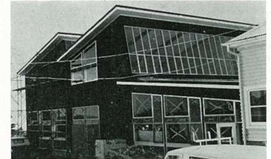
The new Technical Block takes shape.
