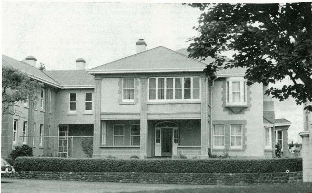
The Hostel warden will reside on the upper floor while the single tutors and senior pupils will use the downstairs rooms.
