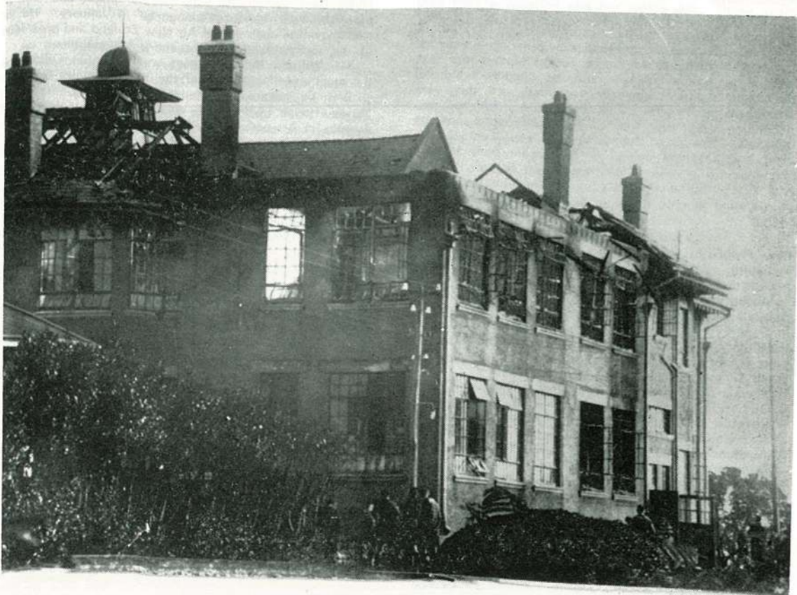
FIRE IN THE OLD BLOCK, 1926
