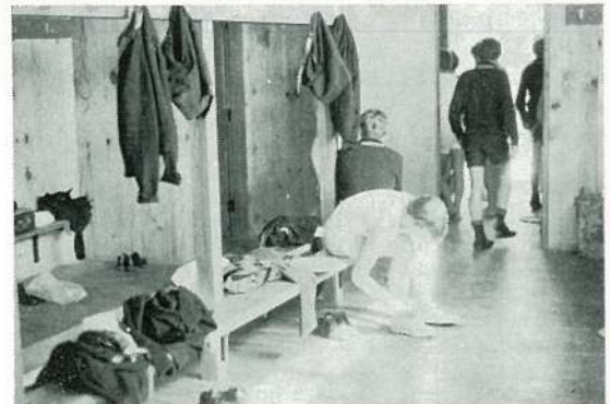
New Gymnasium Changing Room
