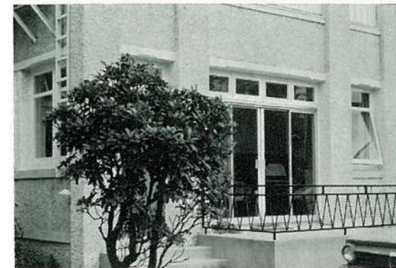
Carrington House—New Entrance
