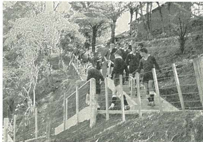
THE NEW STEPS TO THE GULLY IN USE
