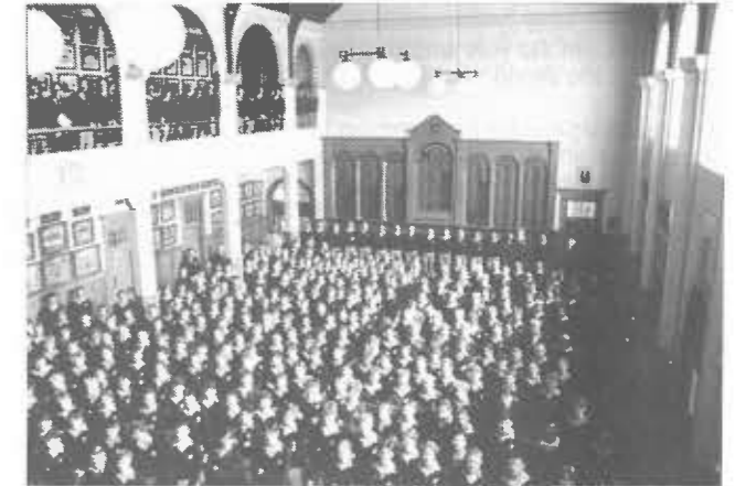
The school assembled in the newly renovated Pridham Hall.
