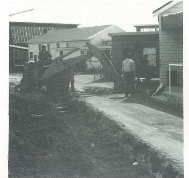
Much construction going on in the early months of the year
