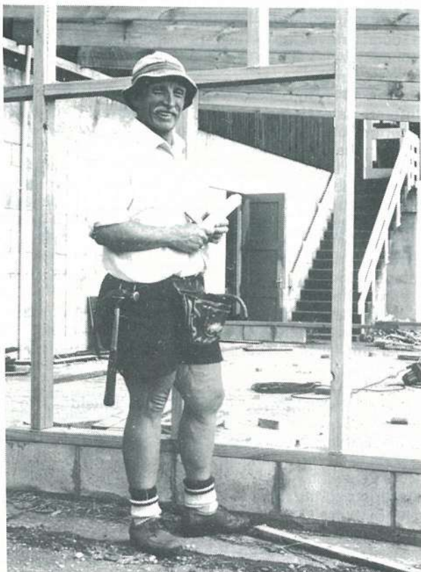
Master builder — M. Grimwood framed by the new Engineering Project Shop
