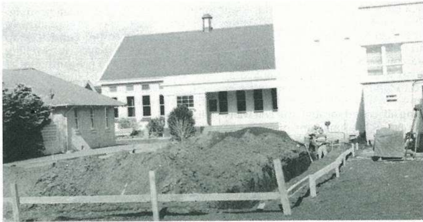
Site of the new Laboratories
