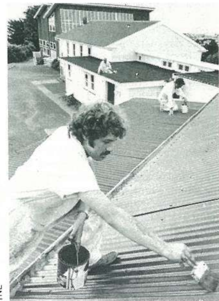
Repainting the Woodwork Block
