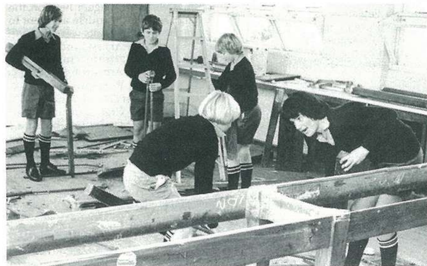
Third formers demolishing the inside of an old laboratory
