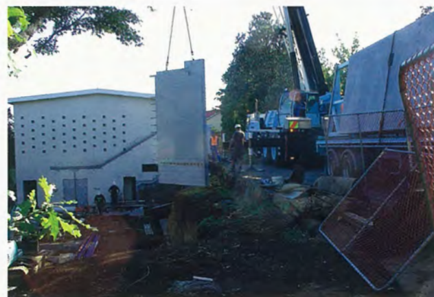
CONSTRUCTION BEGINS ON THE NEW MEMORIAL BLOCK EXTENSION
